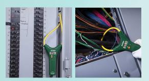
Flexible clamp jaw easily wraps around bus bars and cable bundles that may be difficult to access with regular clamp meters. The thin 7.5mm cable diameter easily fits into tight spaces. Choose between a 10" (25.4cm) or 18" (45.7cm) cable clamp length to accommodate your application needs.
